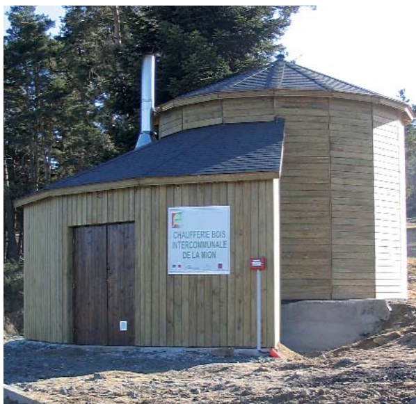
Chaufferie bois - Mazet Saint-Voy
